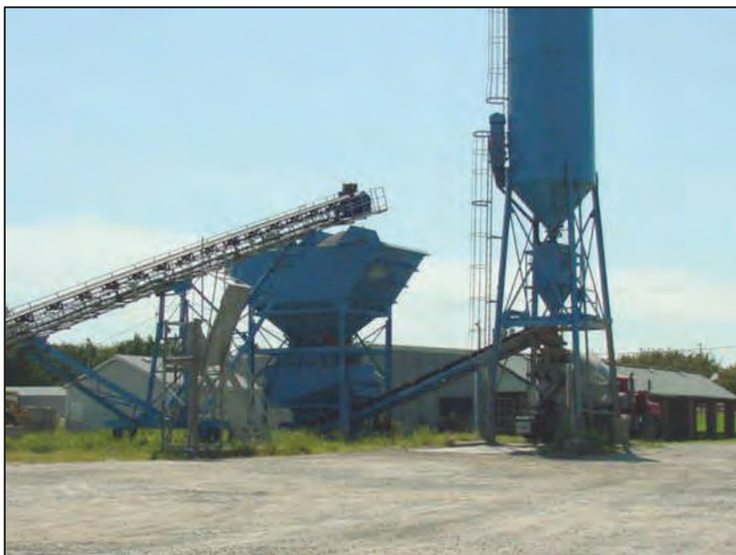
Concrete manufacturing plant components
