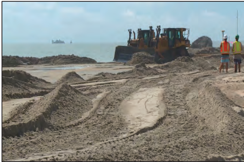
Beach nourishment work in Buxton
